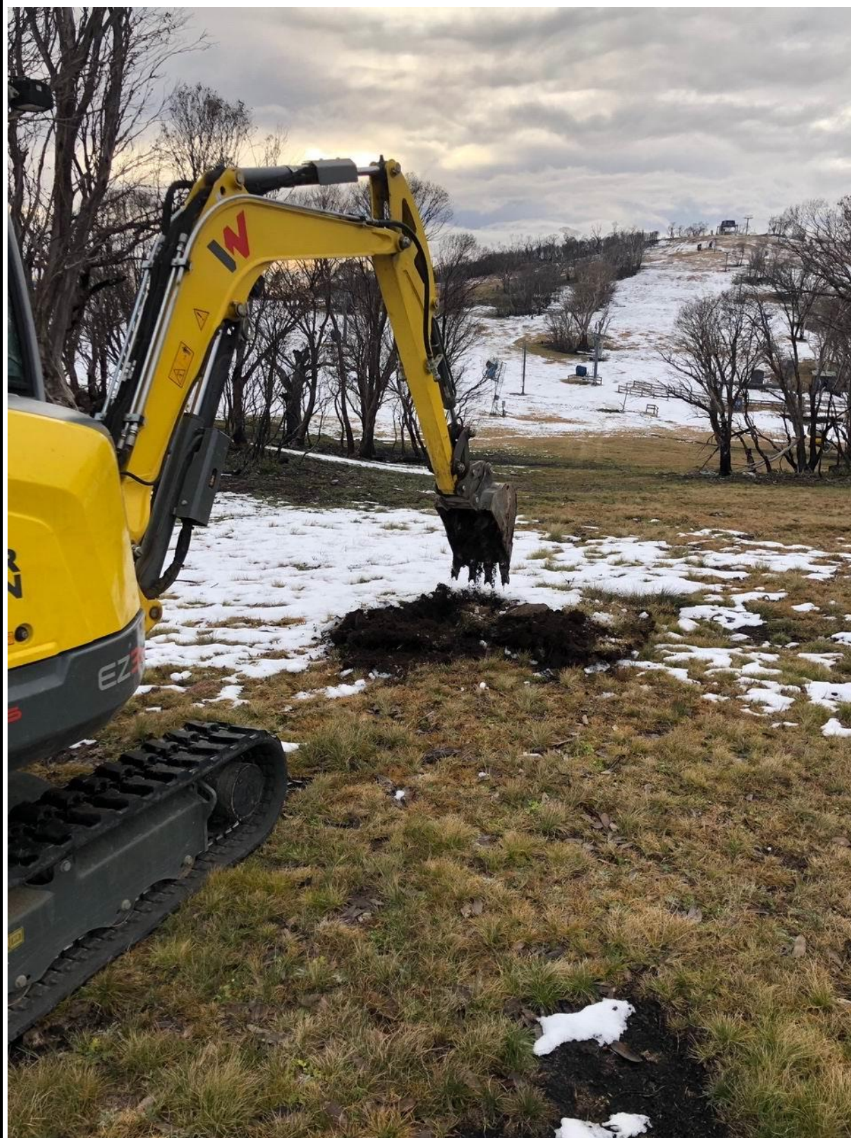
Photo 7 – 10/7/2020 – View of test pit 3T being excavated.
